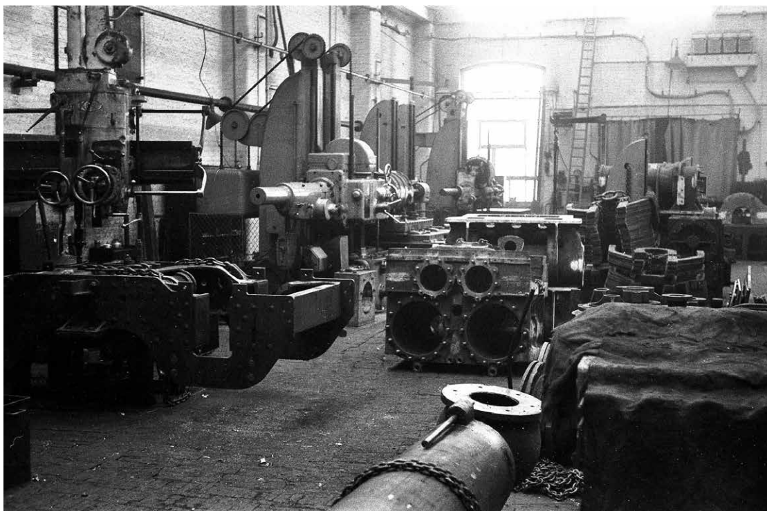
◀ The large machine bay of the Machine Shop in 1960, with horizontal boring machines on the left and new cylinders in the centre
